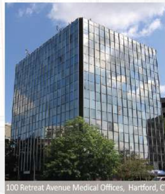
100 Retreat Avenue Medical Offices, Hartford, CT
